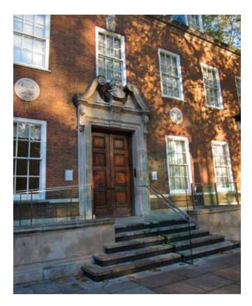
Left: The Foundling Museum, London A ramp to one side of the entrance sits behind an existing wall. The new central handrail to the steps allows for left and right-hand use.
